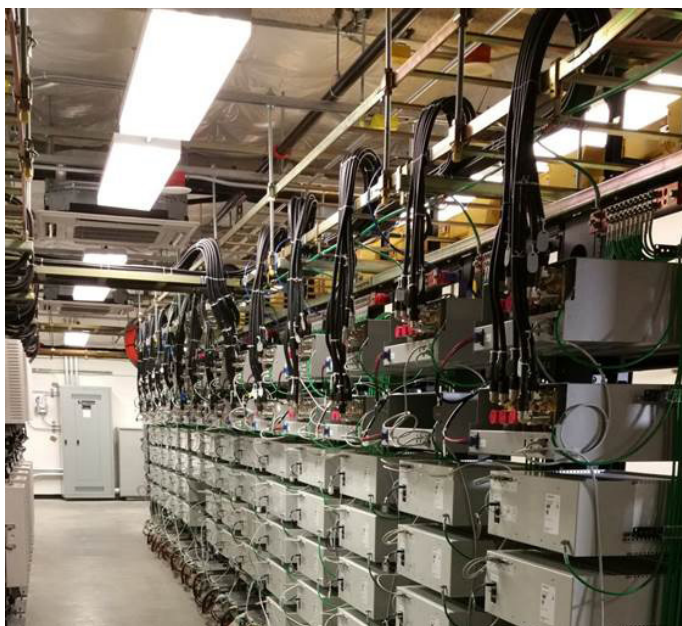
Figure 5. DAS radio headend
